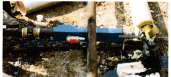
Operator installed a 4" Kinetic Cell.
