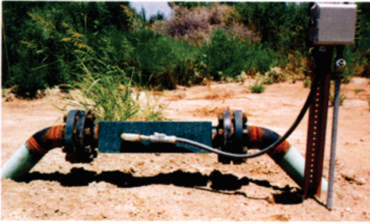
4" Kinetic Cell installed on a 4.7-mile pipeline, operator eliminated chemicals, disposal and maintenance, and reduced paraffin to a trace.
