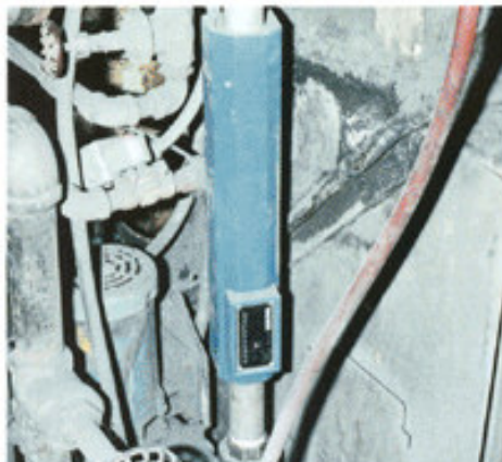
Ener-Tec, Linear Kinetic Cell 1 1/2" 304 stainless steel. Application: cooling tower.
